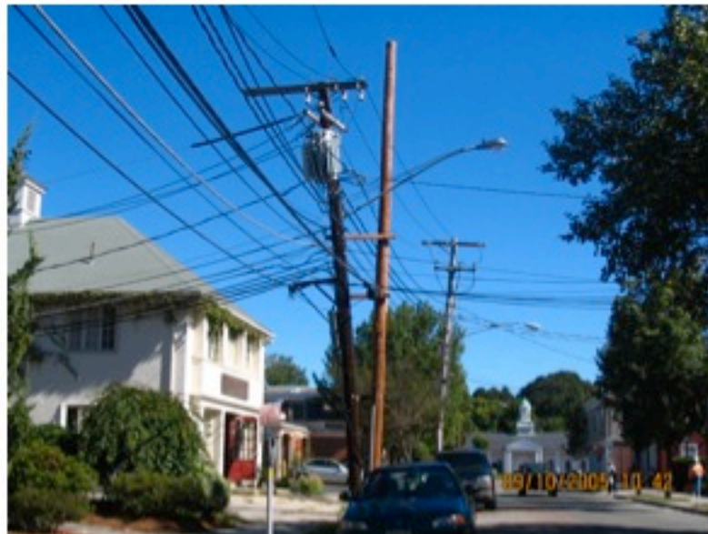
Lexington, NStar : double pole on Muzzey St
